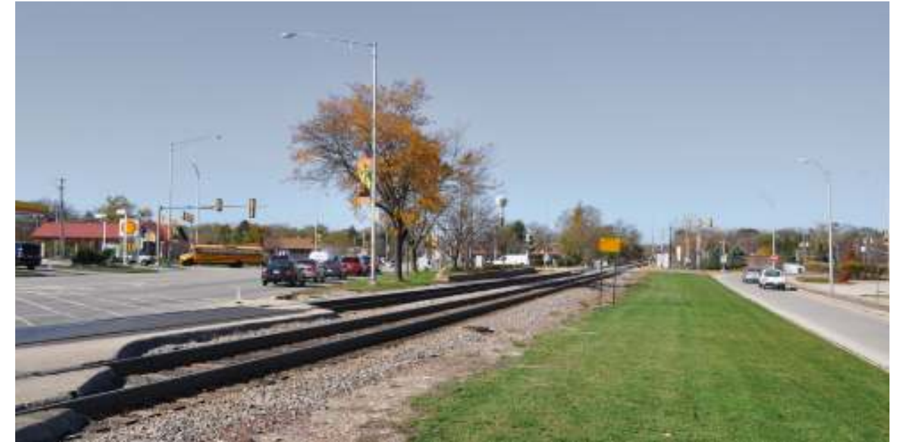
View or rail parkway between Irving Park Rd and Front St before planting
